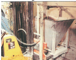
Batching on the Move
