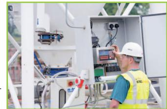
The 1310 indicator provides two-way communication with Head Office via a GSM modem:
